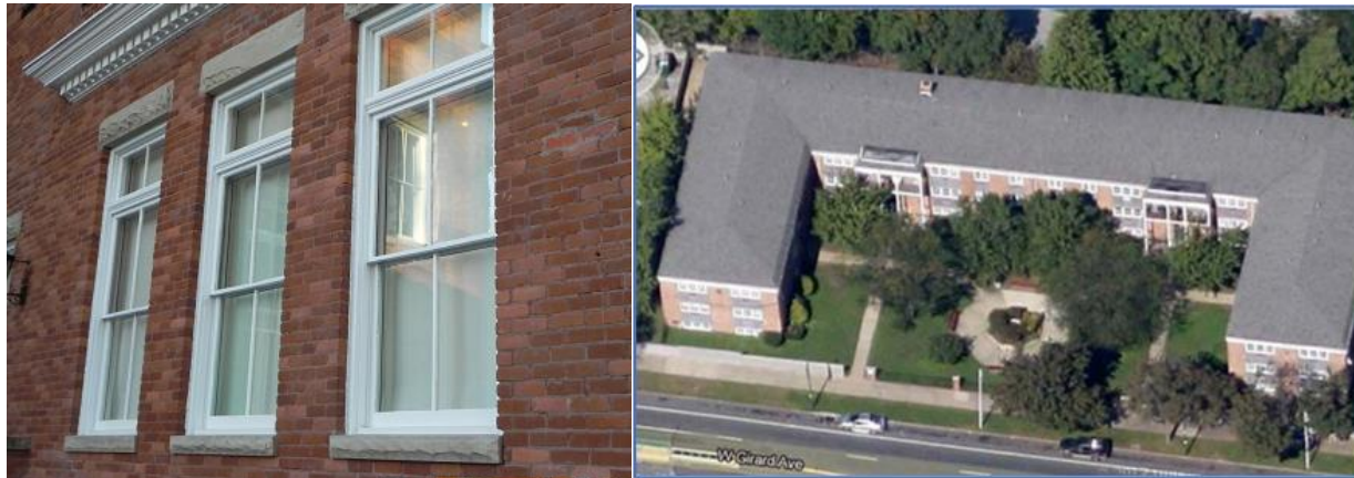
Figure 3. Philadelphia multi-family apartment building with installed low-e storm windows. Source: EERE 2013.
