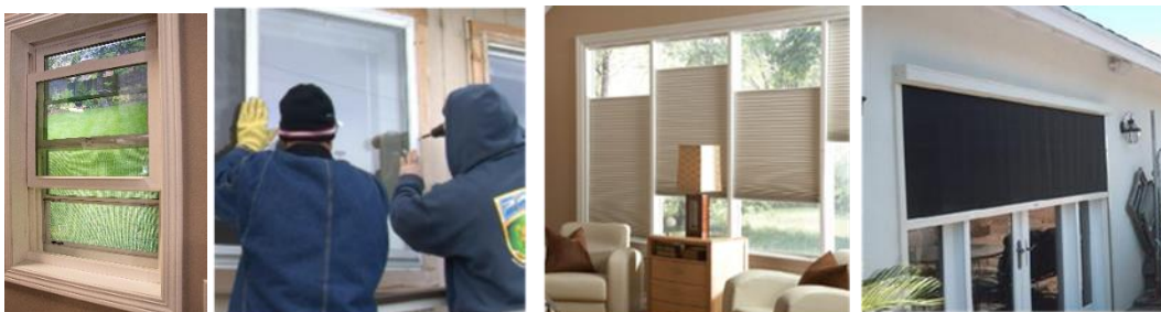
Figure 1. Window attachment retrofits (from left to right) interior operable storm window, exterior low-e storm window, insulating cellular shades, and exterior shades. Source: PNNL, AERC.
