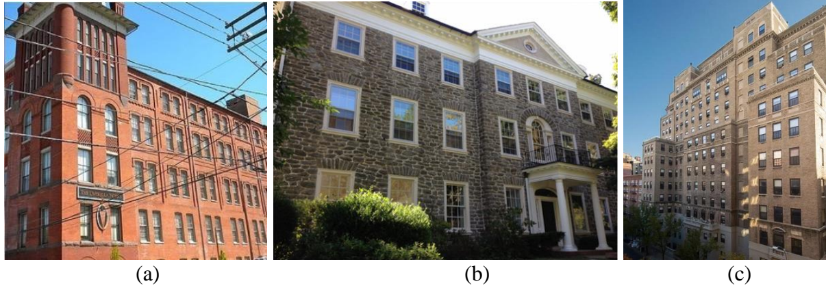
Figure 5. Examples of low-e storm windows on historic multi-family upgrades. (a) 1892 Umbrella Works, Lancaster PA - adaptive reuse to apartments, interior low-e panels. (b) Wissahickon Avenue Apartments, Chestnut Hill, PA - exterior low-e storm windows. (c) 1929 French Apartments, New York City, NY - interior operable low-e panels. Photos courtesy of QuantaPanel.
